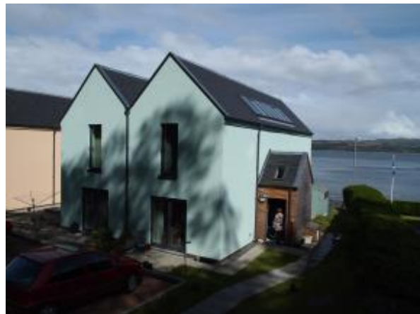
Figure 2 - Dunoon Passive House – Note Solar Thermal Panel Installation
