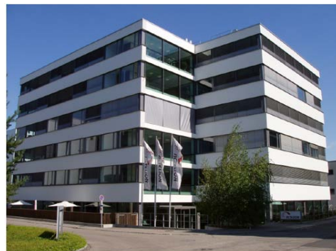
Figure 1 View of the target building from the south
