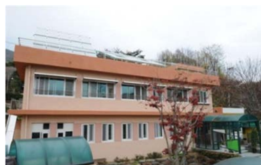
Figure 14 Outside view of the existing building
