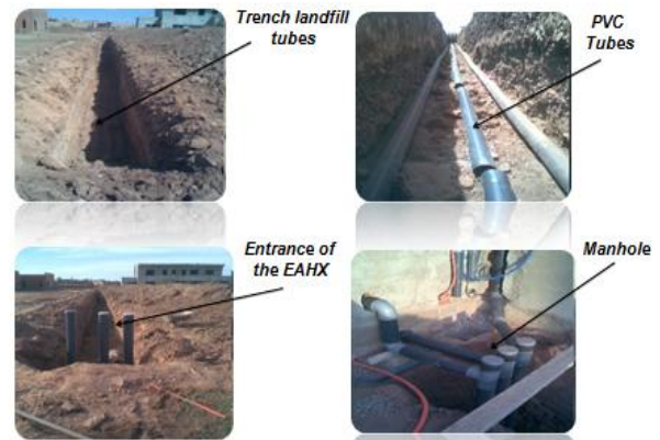
Figure 2: Implementation details of the EAHX.
