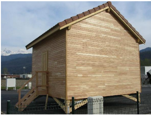
Figure 1 Photograph of the north and east of the experimental house
