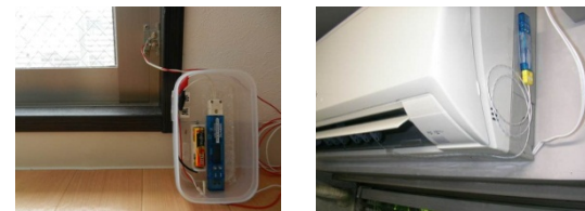
(a) Window (b) Air conditioner
