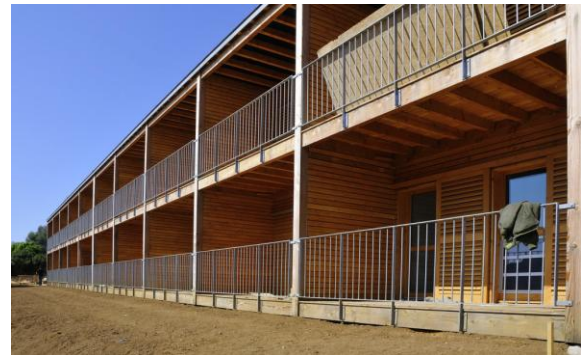
Figure 1: East facade of "Le Charpak" building
