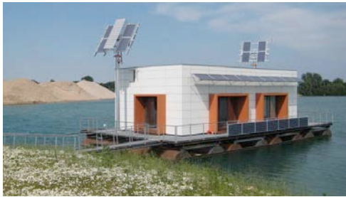
Figure 1 Photo of survey building
