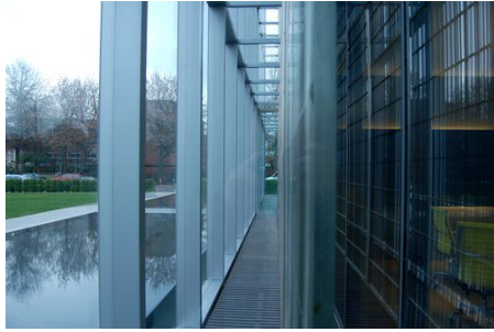
Figure 6. View towards double skin façade on the first floor
