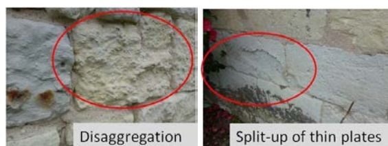
Figure 2 Disaggregation of Tuffeau stone (left) and split-up of thin plates of Tuffeau stone (right).
