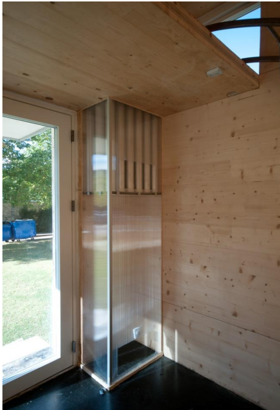
Figure 3 The naturally ventilated air-to-air heat exchanger
