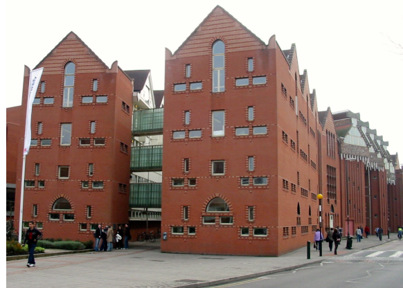
Figure 1: The Queens Building
