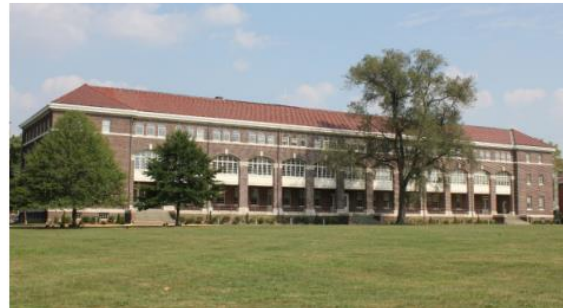
Figure 9 Building 101 in Philadelphia, PA
