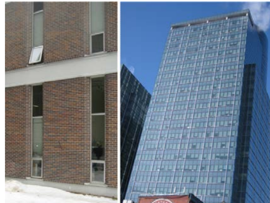
Figure 2: Examples of unintended results of actions taken by occupants who were presumably uncomfortable: open window in winter (right) and high shade occlusion level (left)
