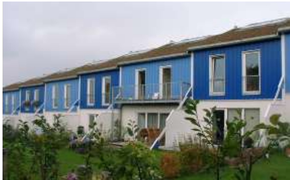
Figure 3 South facades of the Hannover Terraces(Feist et al. 2001)
