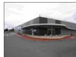
Figure 1 North facade – Est – Entrance
