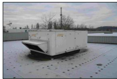
Figure 2 Screw heads appearing on the roof
