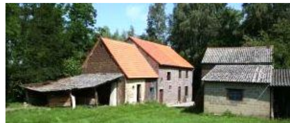
Figure 8 – Picture of the house in project ZEHR (Zero Energy House Renovation) (Peeters & Mols, 2012)
