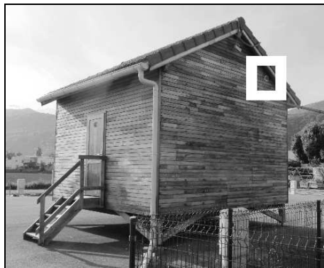
Fig. 1: Picture of the experimental set up (western and northern sides) with location of the ventilation opening
