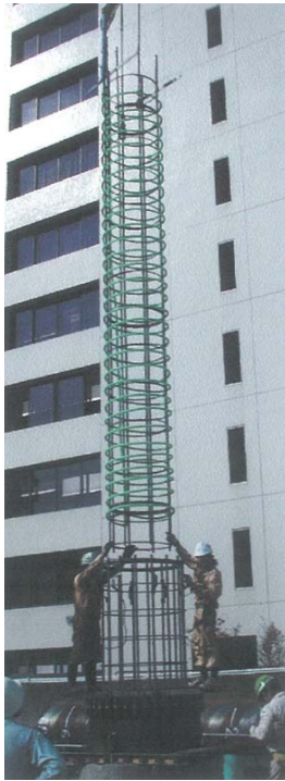
Figure 3 Construction of a pile
