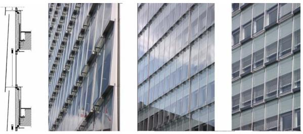
*Fig.* 14 – '*staggered shaft façade*', *implemented* 2002
