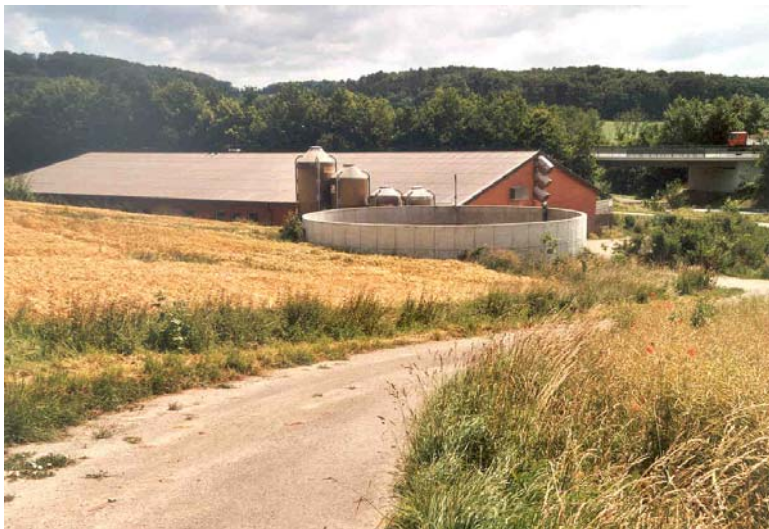
Figure 6 Realized removal of the air of a piggyery on the gable side. Side wall fans blow out stable air on the leeward ground, which has an effect like a baffle. Mechanically induced turbulences are produced. This effect is supported by a wall of earth in front of the gable. The immission of odour 200 m behind the end of the animal house (left side) is lower in comparison with the situation of emission by stacks on the roof.
