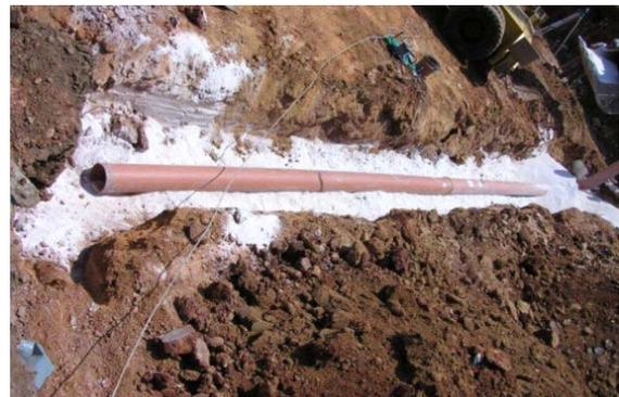
Figure 5: Placement of a pipe into the ground using sand to improve thermal contact between the pipe and the soil
