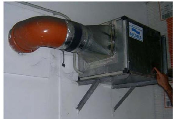
Figure 9: Point where the air from the earth tube is introduced in the building
