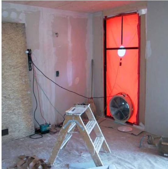
Figure 5: Minneapolis blower door
