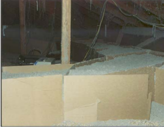
Blown –in insulation with cardboard forms
