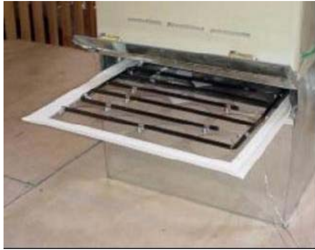
Flow plate used to measure air handler flows (Paul Francisco, ECOTOPE, Inc.)
