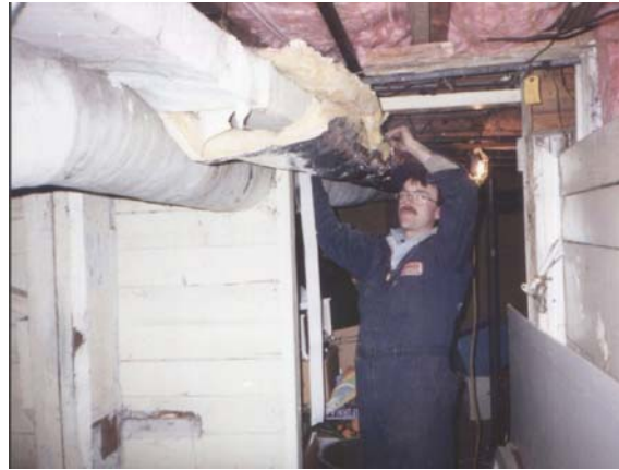
Installing Duct Wrap
