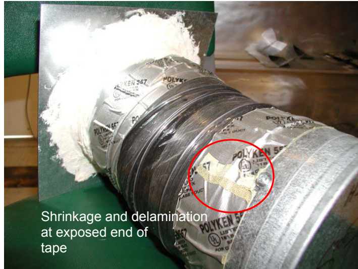
Figure 12. Shrinkage and delamination among the unclamped specimens (after 5 months of aging)
