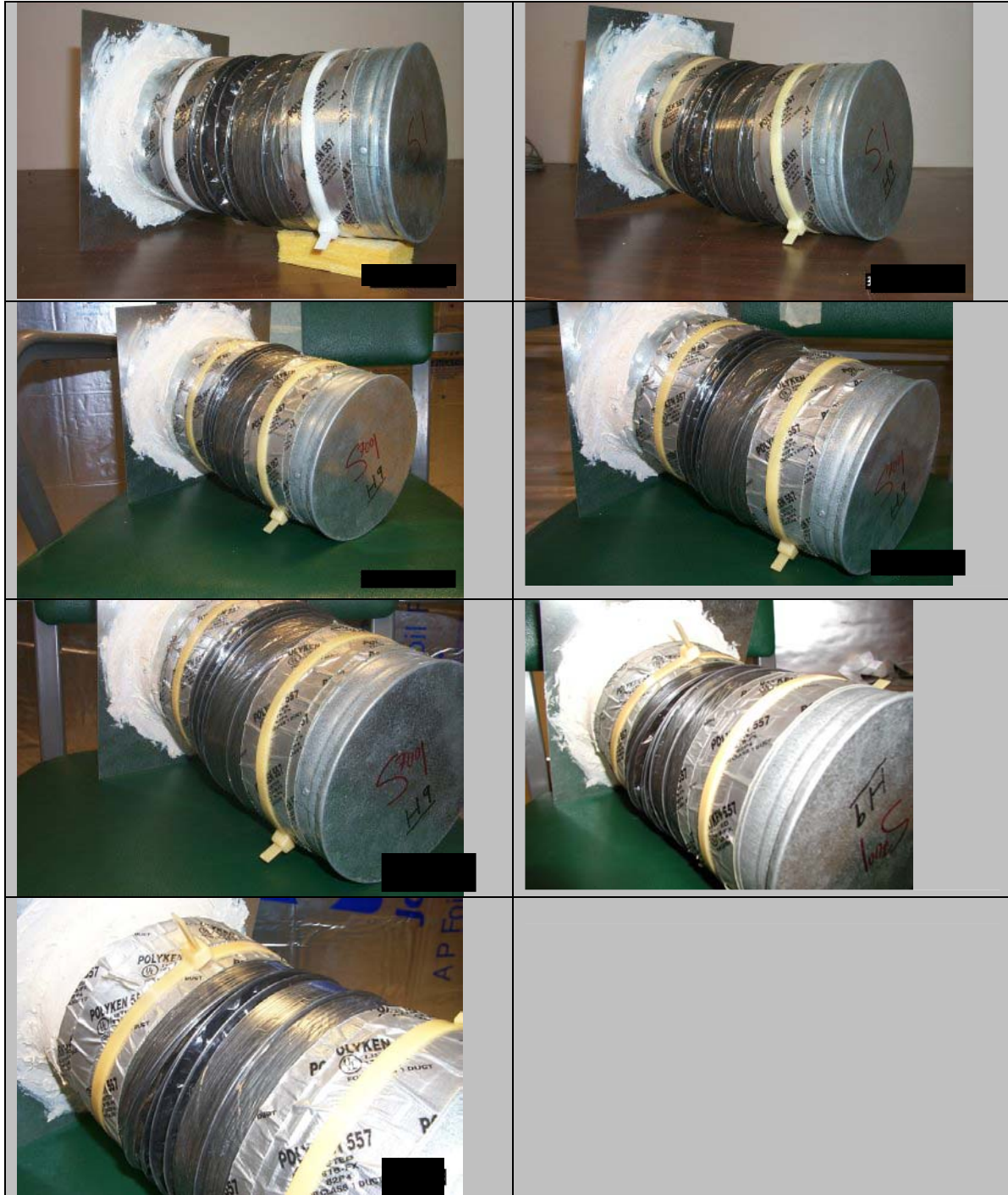
Figure 11. Deterioration of flexible duct core-to-sheet metal collar joint during the six months of the aging test.
