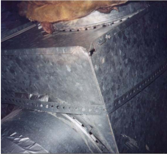
Figure 2 - Example of collar-to-plenum connections on a system where the tape sealant has fallen off, and a collection of collar-to-plenum test samples from LBNL.
