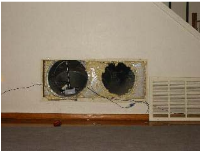
Figure 16. Duct sealing of downstairs return using foam. [the sensor that is visible is a relative humidity sensor, there is also a temperature sensor in the duct].
