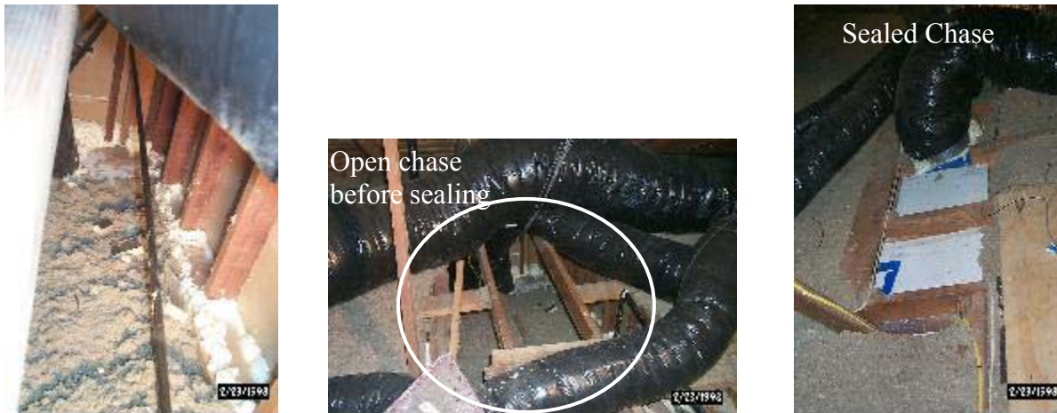
Figure 6. Sealing cavities connecting the house to the attic. Foam is a useful sealing tool for small holes and cracks at building component intersections (left). Duct board insulation can be used to block off large open areas (center and right)
