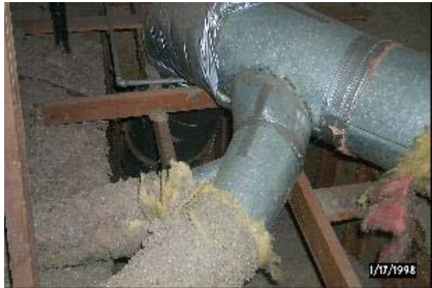
Figure 5(c). Existing supply duct run from garage to attic showing large openings in attic floor plane [above stairway dropped ceiling].
