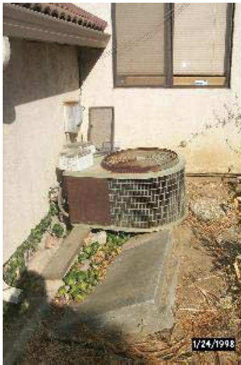
Figure 4. Existing AC condensing unit outside near rear of garage showing poor condition of unit [heavily corroded sheet metal fasteners and significant dirt/dust accumulation blocking flow into coil] and subsided slab [stressed refrigerant tubing and subsequent leakage of refrigerant].
