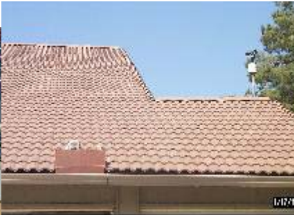
Photo B.3. Location of pyranometers on roof with wind tower in background
