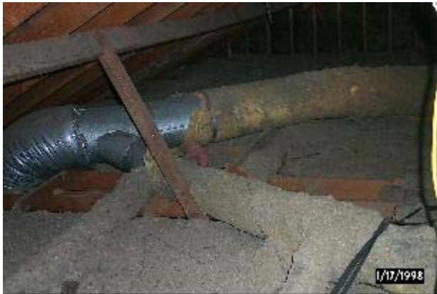
Figure 5(c). Existing supply duct run from garage to attic showing large openings in attic floor plane [above stairway dropped ceiling].
