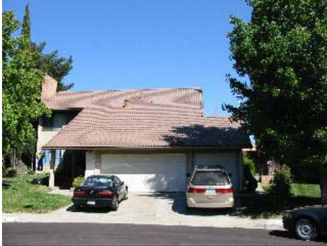
Figure 2(a). Exterior front view of Concord test residence.
