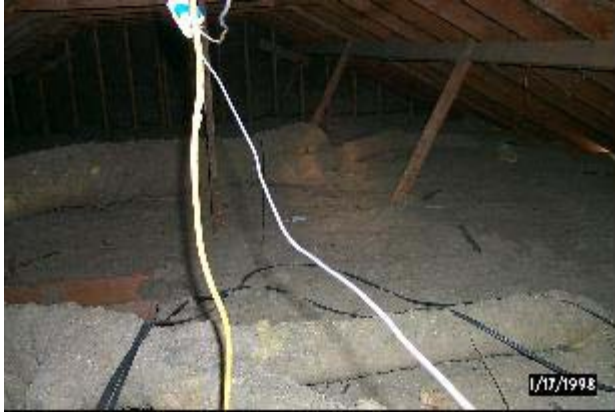
Figure 5(a). Existing attic floor showing insulated metal ducts and insulation coverage.
