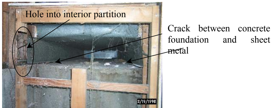
Figure 5(d). Existing return cavity between foundation and lower level floor.
