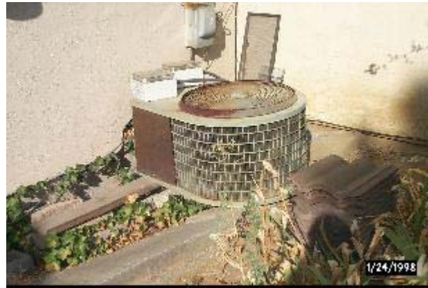
Figure 4. Existing AC condensing unit outside near rear of garage showing poor condition of unit [heavily corroded sheet metal fasteners and significant dirt/dust accumulation blocking flow into coil] and subsided slab [stressed refrigerant tubing and subsequent leakage of refrigerant].
