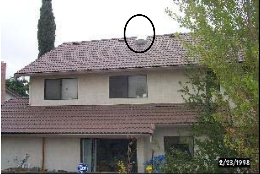
Figure 10. Installed roof mounted economizer vent.
