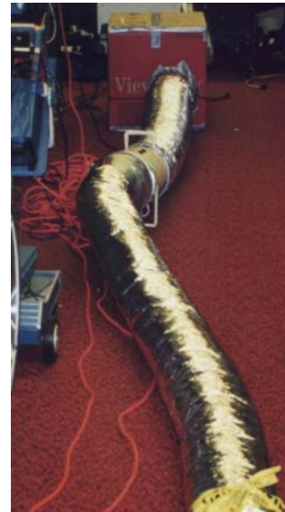
Figure 7. Bends in the duct radiatively isolating the duct air temperature sensors from the heating elements.
