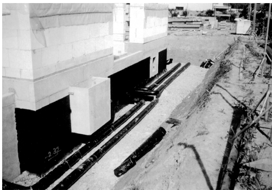
Figure 6.8 Ground Heat Ducts (Courtesy EMPA Switzerland)
