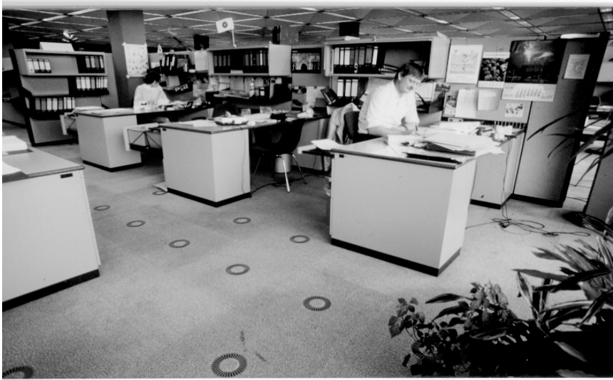
Figure 5.12 Balanced ‘Displacement’ Ventilation (office) (Courtesy FGK, Germany)
