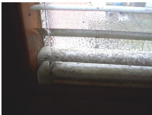
Figure 2: Condensate on glazing internal surface, and mould on internal blinds.
