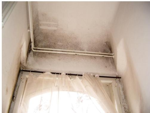
Figure 4: Mould growth on the bathroom ceiling, heating turned off, poor ventilation.
