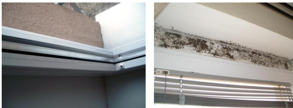
Figure 3: Left, new energy efficient and airtight windows in an uninsulated wall. Right, consequences of constant ventilation with window in an inclined position.
