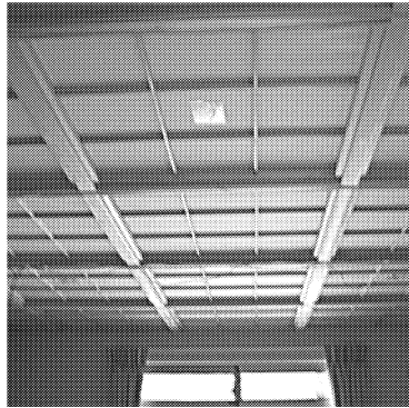
Figure 1: The ceiling surface made of “Washi” and wooden frameworks
