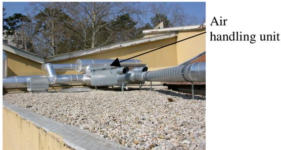
Figure 1 : Air handling unit on terrace roof
