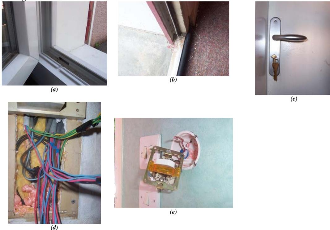
Figure 1. Examples of refurbishment measures. (a) replacement of windows. (b) Replacement of undercut joint and joint around the opening. (c) Replacement of the garage lock. (d) Injection of insulation foam to close the passageways to the air gap in the wall. (e) Insulation foam behind the plug boxes in cold walls.
