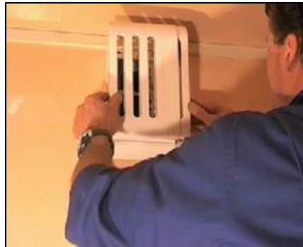
Figure 5 : Position of the grille face.
