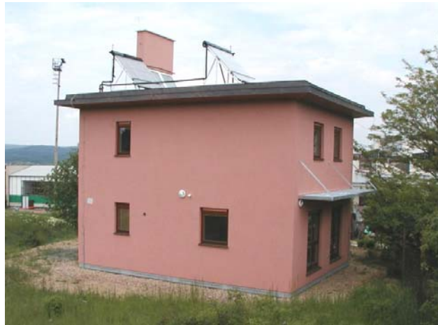
Fig. 7 Experimental house with hybrid ventilation
