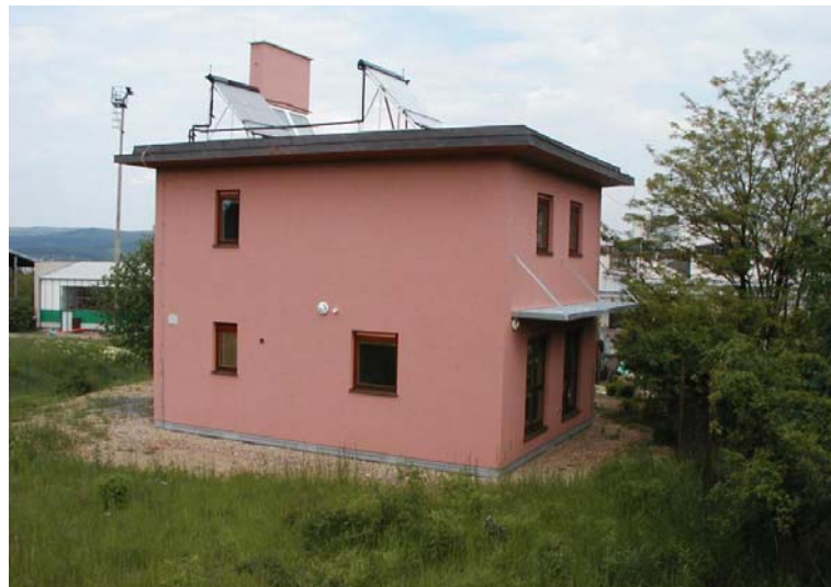
Fig. 1 Demonstration house with hybrid ventilation
