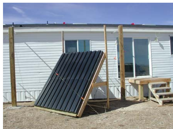
Figure 2. SolarWall system on manufactured home, Arlington, WY, Winter 2003.
