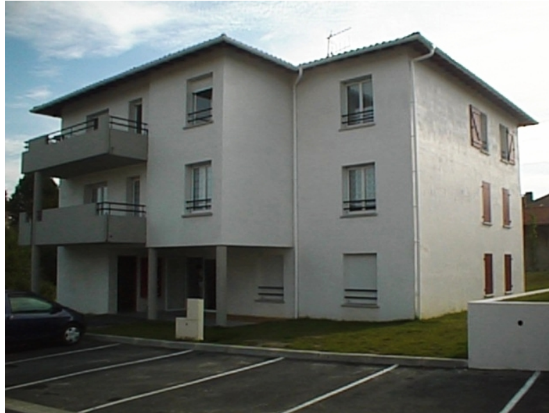
Figure 2: South wall from the building
