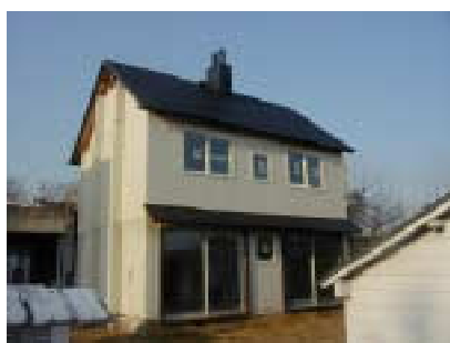
Figure 1: The full-scale test house
