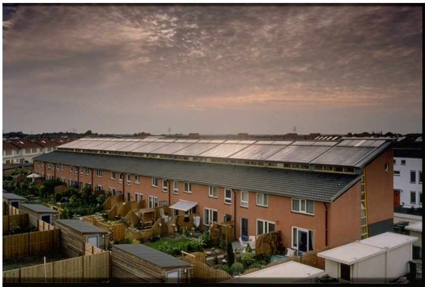
Figure 1. Roof integrated solar thermal and electrical collectors
