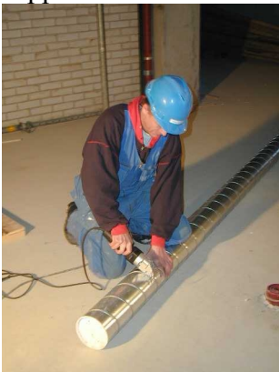
Figure 2. (Left) New cleaner cutting methods in practice. See also the capped end of the duct.
