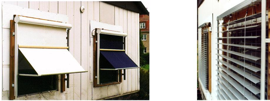
Figure 1: Twin-boxes equipped with italian awnings (left), and external venetian blinds (right).
