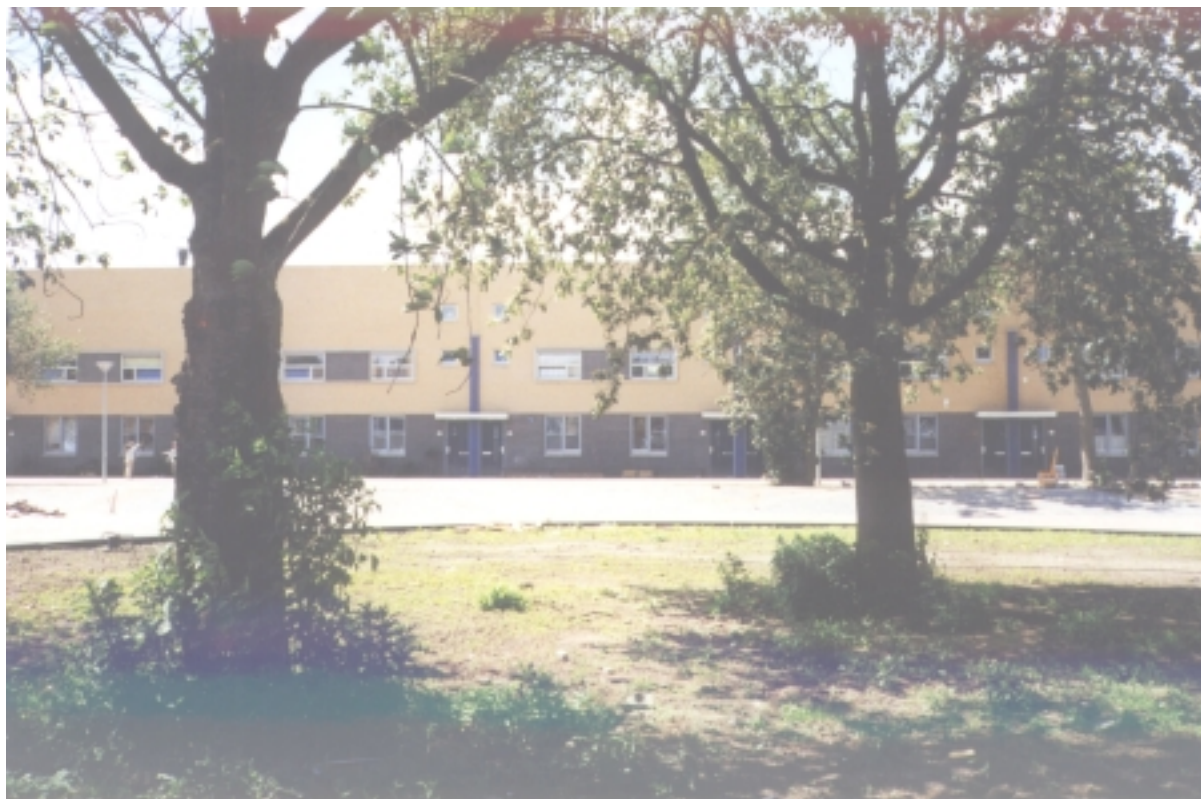
Figure 1 View of dwellings, north facade
