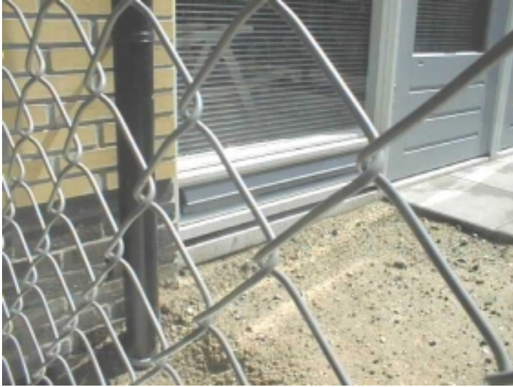
Figure 3 Self-regulating ventilation duct at bottom of sun room
