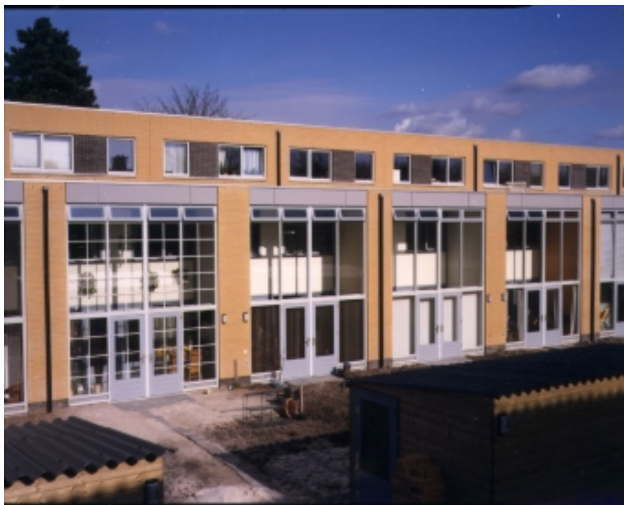
Figure 2 View of the sunrooms
