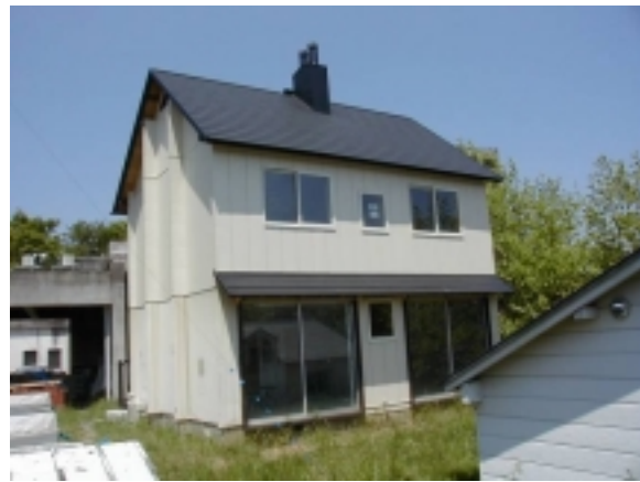
Photo 1 A full-scale test house
