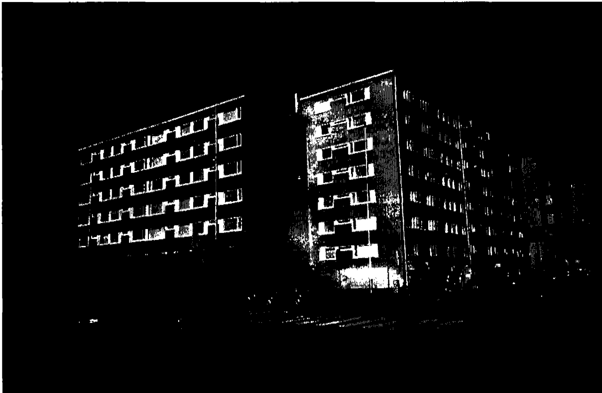
Figure 1. Building in summer 1998 after the new windows have been installed.
