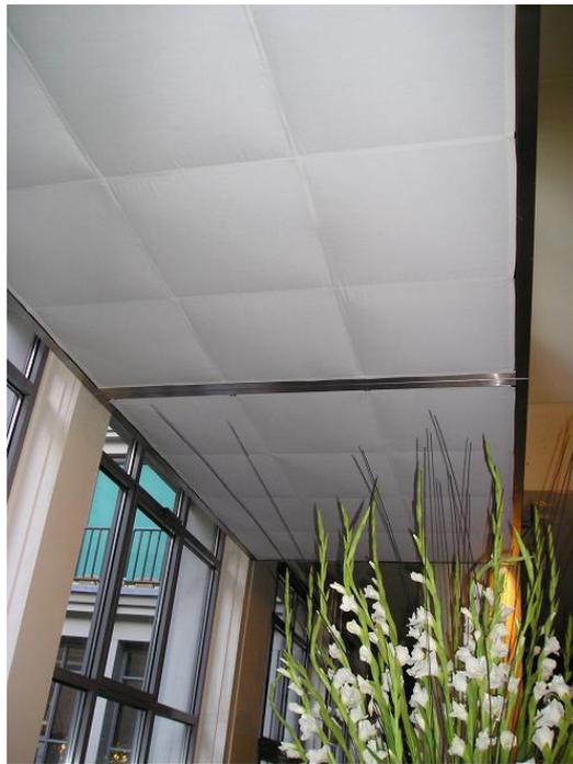
Figure 13: “down flow” cloth fastened with Velcro in segments of 0.6 by 0.6 m<sup>2</sup>.
