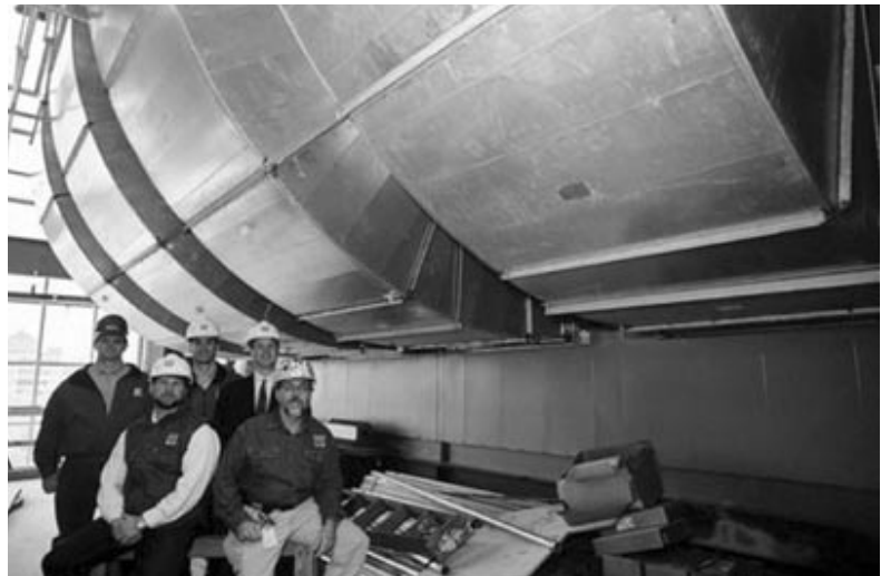
The design and planning team in the mechanical penthouse of Building 50, a new research laboratory in the National Institutes of Health campus in Bethesda, Maryland. Behind the team are supply ducts for the building's air handler.
