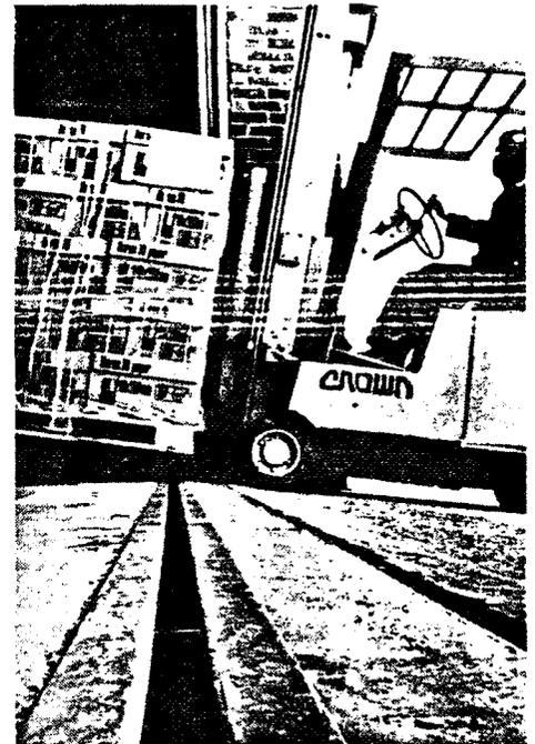
Above. The angled slot on an ambient air curtain at Rank Xerox distribution centre, Slough, projects the air stream upwards forming a protective barrier over the doorway. (Bahco)
