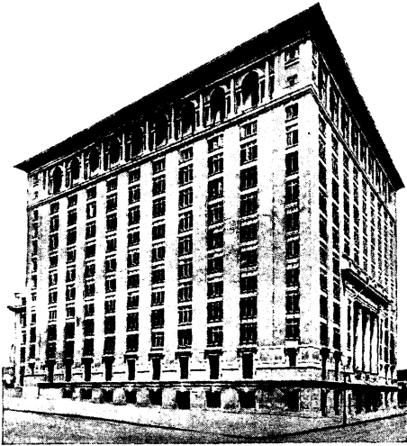
FIG. 1. GRAND CENTRAL PALACE BUILDING, LEXINGTON AVE. AT 46TH ST., NEW YORK, N. Y.
