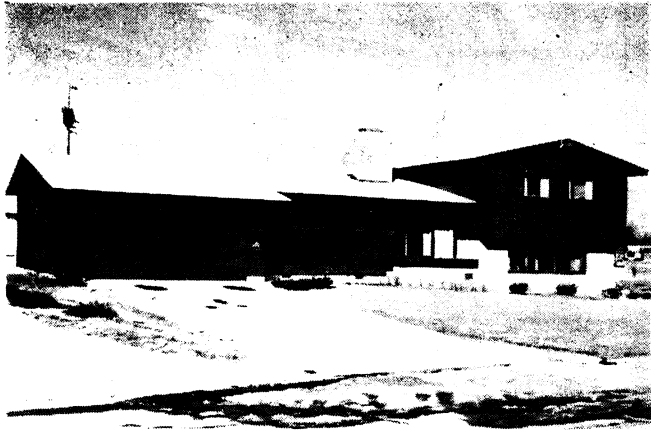
Fig. 1 Exterior view of I-B-R Hydronic Research House
