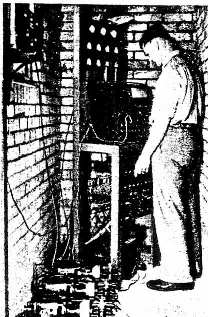
Fig. 8—Recorder hut containing remote controls
