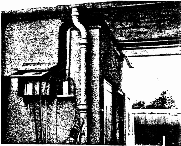
Fig. 6—Copper tubes used for introducing tracer gas and extracting air samples
